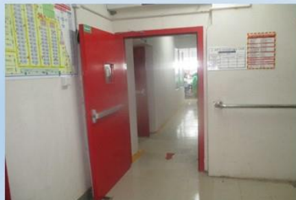
Fire Door Installation
