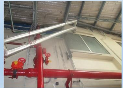
Fire Stand Pipe Installation
